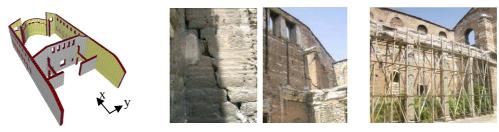
(a) (b) (c) Figure 3 : The monastery in 3D (a); Cracks-main wall and supporting column (b); the collonade and the architraves (c)
